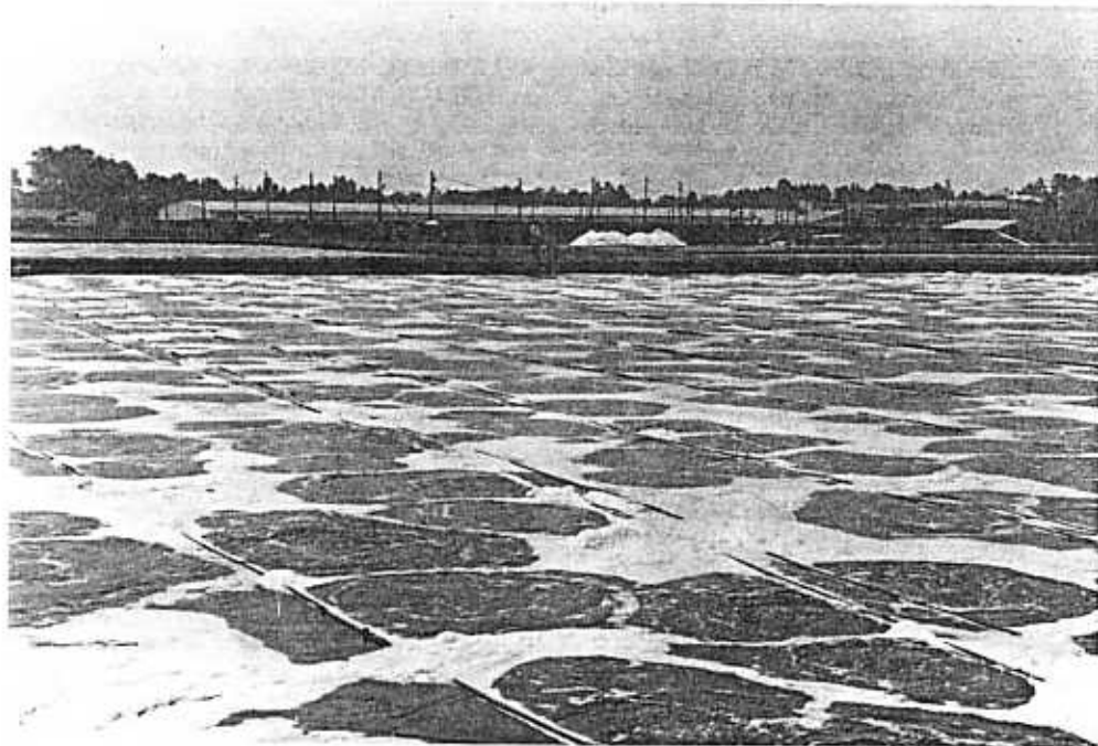
FIGURE 11. Waste treatment lagoon at a pickle-processing plant.
